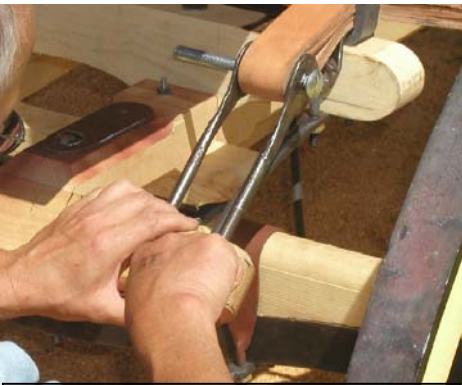
Tightening the thorough braces
