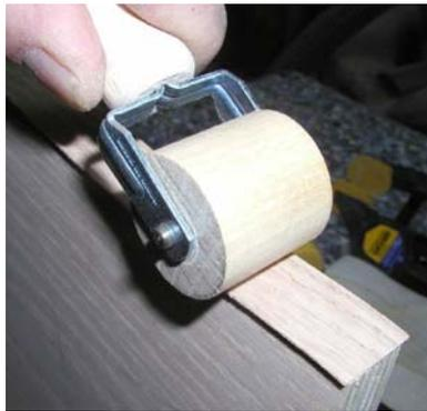
**Pressure Sensitive:** I expected the adhesive to be unforgiving during positioning. No so, as long as you don't press it down. I expected to need a large, two handed roller to generate enough pressure. This one pictured worked quite well and is very inexpensive.
