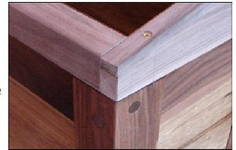
The last part of the end caps is the end cap cover, 1/4 inch thick and 1 inch wide. They get glued to the previously attached spacer. In the photo the end panel cover was bent to shape after soaking in hot water.
