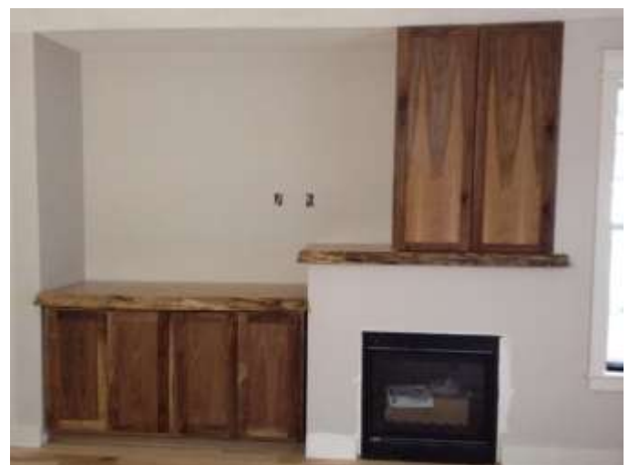
Sherwood house cabinets installed
